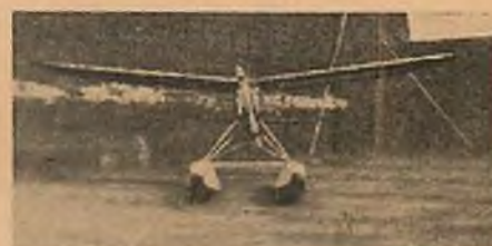
Paul Broccard of New York built this gas-powered seaplane, weighing 6 pounds complete with G. H. Q. engine and pontoons.
