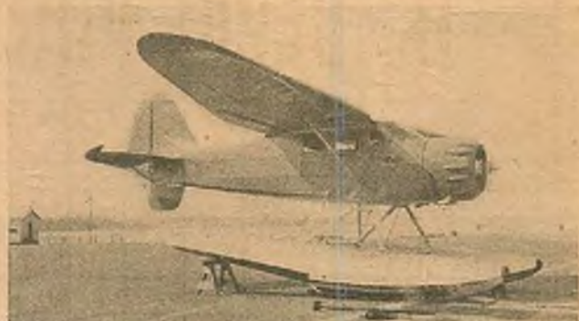
Stinson Reliant, powered by 320 h.p. Wright Whirlwind, is first of 1937 series to be equipped with floats. Rounded windshield and new-type cowl are recent modifications—small fin on seaplane only.
