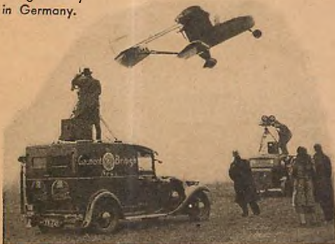
The Dutch version of a foolproof plane—it crashed on test flight—is equipped with a 40 h.p. pusher engine.
