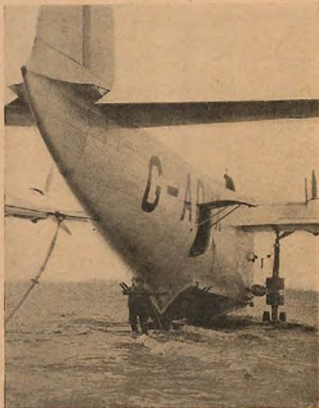
This striking view of the English flying boat Cassiopeia, being drawn from the water for overhaul, clearly reveals the flowing hull lines of the giant.
