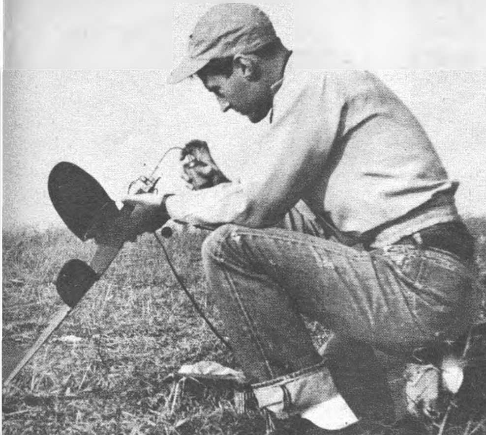
The designer primes the engine of his duo-mono before starting. Developed through a series of models, it is extremely stable, especially in the stalls, and is an excellent windy weather performer.
