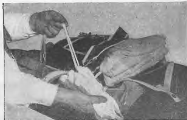
11 The pilot 'chute is now collapsed by folding spring ribs together and pulling pilot 'chute shroud lines with hand.
