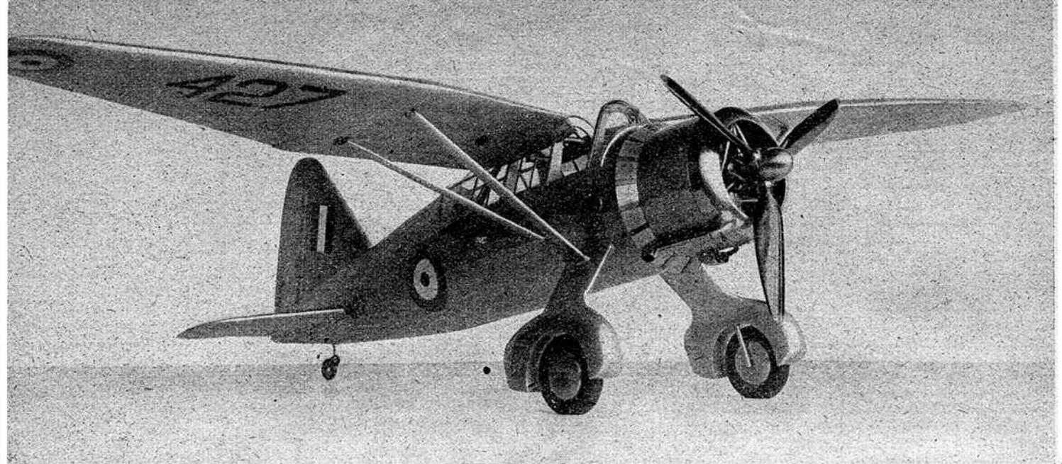
*A 1/10 scale, i.e., 5 ft. span model of the Westland Lysander powered by a 3 c.c. Ohlsson engine. Construction and finish leave nothing to be desired and the builder, Corporal A. Welsberg of the Polish Air Force, is to be congratulated on a magnificent job of work. Details of the model are given below.*
