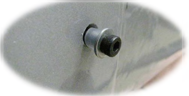
Photo 11: Notice the section of fuel tubing on the bolt that isolates vibration
