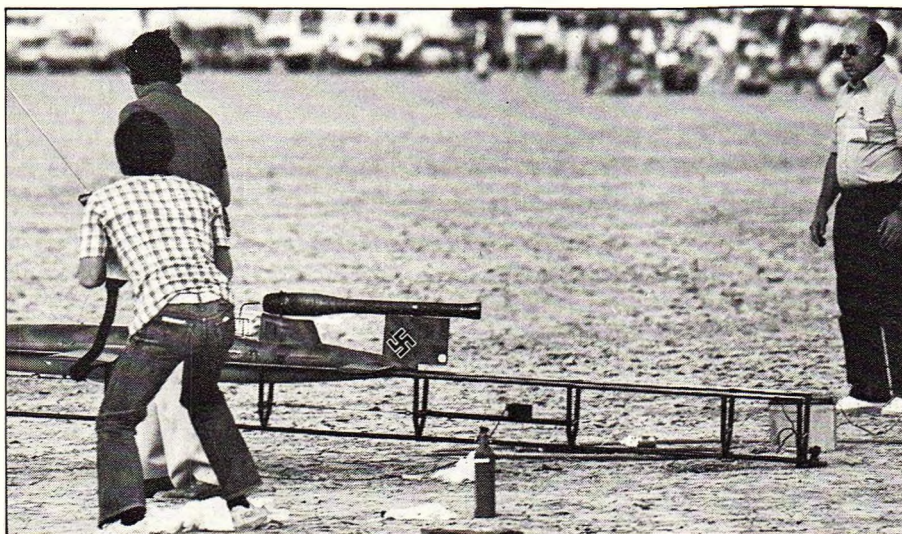
The pulse-jet powered Buzz Bomb, being catapulted off its elaborate launch ramp. The photo clearly shows the bungee cord which helps it get momentum. The jet reaches speeds in excess of 200 mph!
