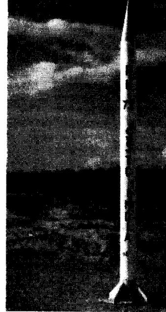
The RH-75—the first of the Rohini series of sounding rockets.
