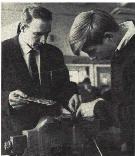
Johnson shows student Wayne Hiatt fine points of safety wiring. Students are taught aircraft construction, hydraulic and electrical systems and maintenance. Student graduates with airframe mechanics license after two years of training.
