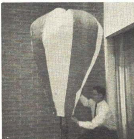
Tin-can furnace is more efficient and inflation easier when sheltered from wind.
