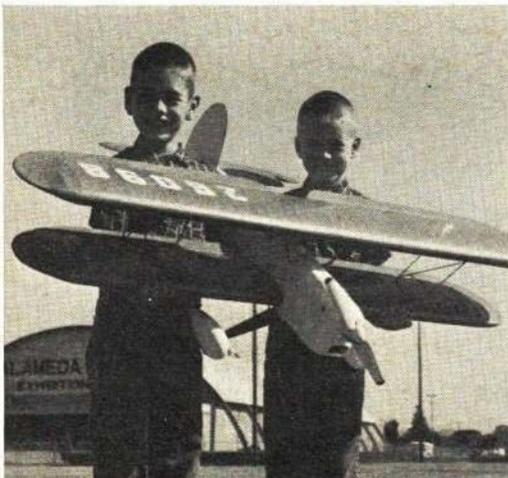
High-lift, high-drag, with big prop, make the biplane fly like a 'copter with rotor facing forward.
