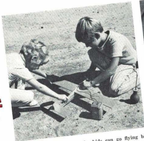
Balsa models are painted with model airplane dope so that the fuel and exhaust do not seep into the wood. Use two coats of clear and two coats of color.
