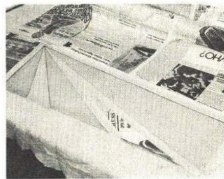
If spraying, completely mask the area to be second color with tape and newspaper.
