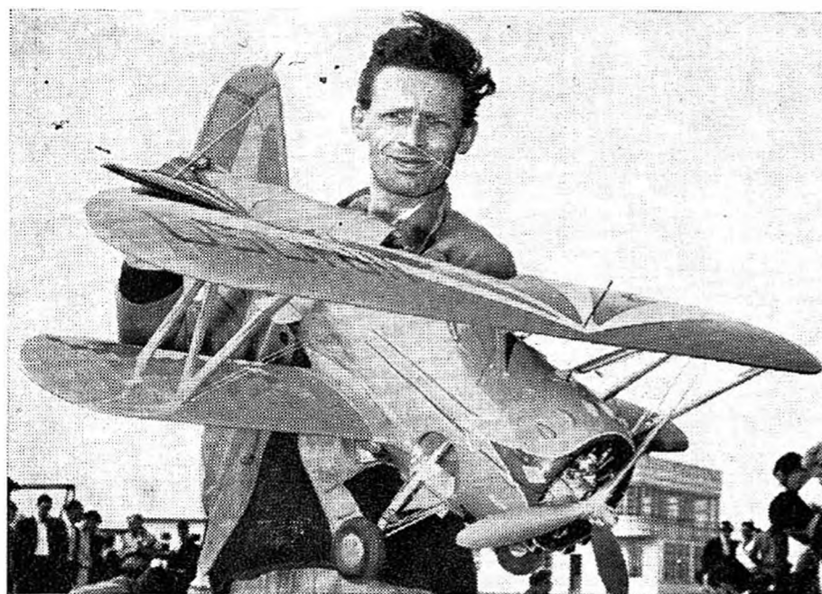
Pete Ball's (Wanstead W'H'K's) magnificent Nats 2nd place control line scale Grumman Gulfhawk with sprung U/C opening luggage hatch, sliding cockpit canopy and scale dummy engine to match the silver foil covered three blade propeller. A Merco 49 R/C lifted and flew this 5½ lb. orange white and blue beauty.
