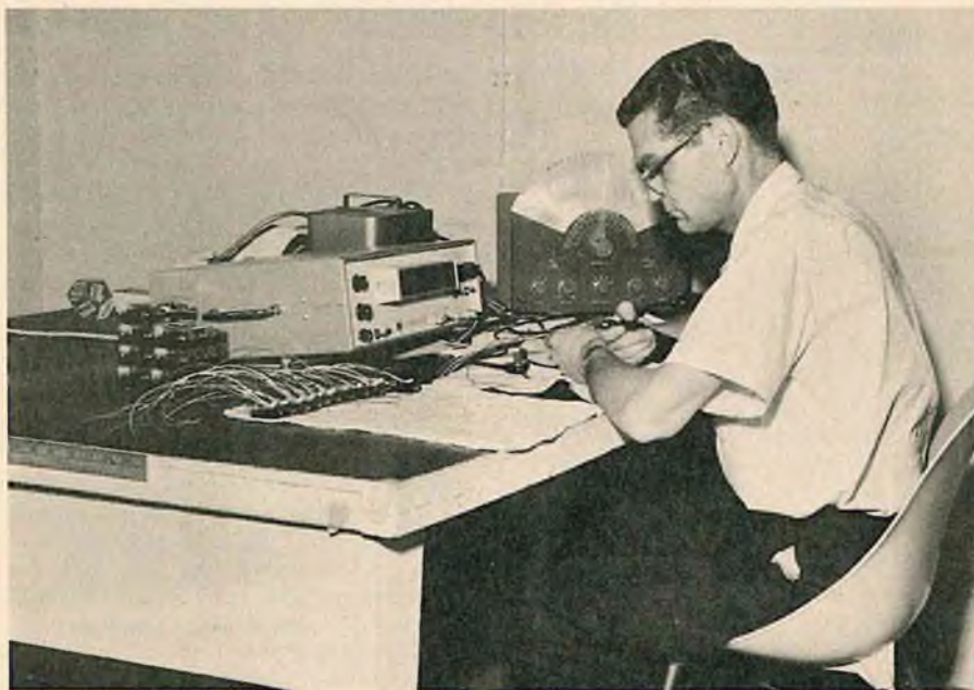
Electronic counter for adjusting reed frequencies to a tolerance of one c.p.s.!
