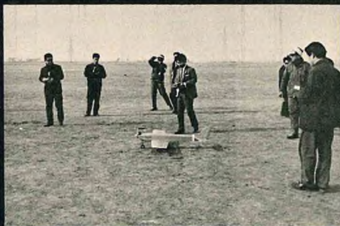
Kando's Bictaire breaks ground on takeoff. A reed ship, it uses 2° dihedral, thick section, and short moments.
