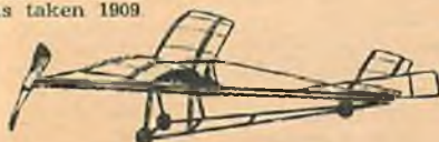
• An experimental racing tractor built by author, flown, '09. Cambered lifting stabilizer.
