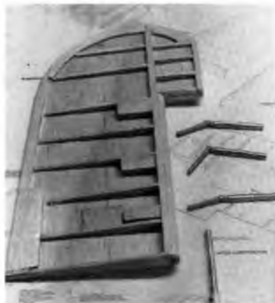
Stab is built in a clever way to duplicate fabric-covered surfaces.
