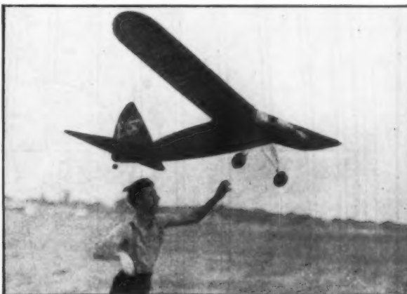
Risky business—Frank Ehling of Jersey City does a little overhead glide testing of his gas job to determine correct balance. Sometimes the model is safely retrieved. The model or its builder must be "good"
