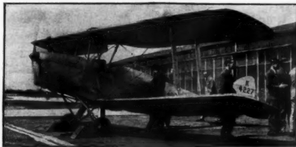
This is Britain's wireless controlled airplane. It flies at 100 m.p.h. and is controlled from the ground
