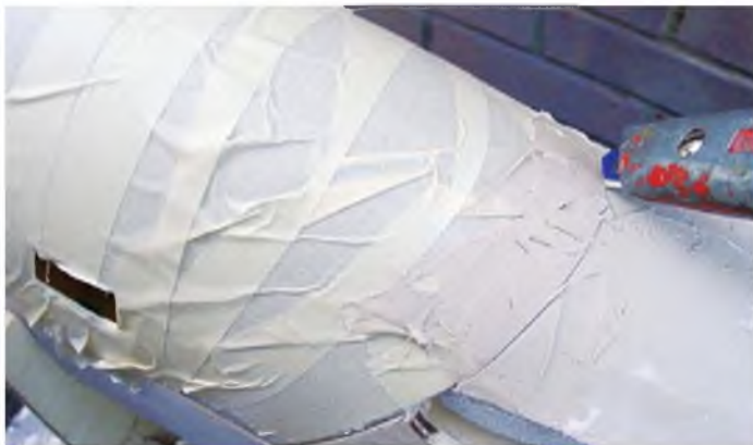
Easing out the joints before the filler gas completely set.
