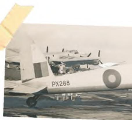
through during 1948, these with a revised tailplane shape and distinctive dorsal fin strake which is the most immediately discernible difference between the two Marks.
